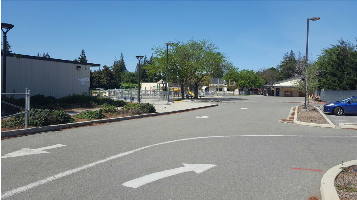
Figure 5: View of Existing Slater School Buildings (to be removed)
