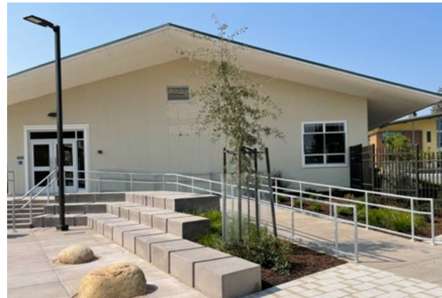
Permeable pavers, La Entrada Middle School, Las Lomitas Elementary School District.
