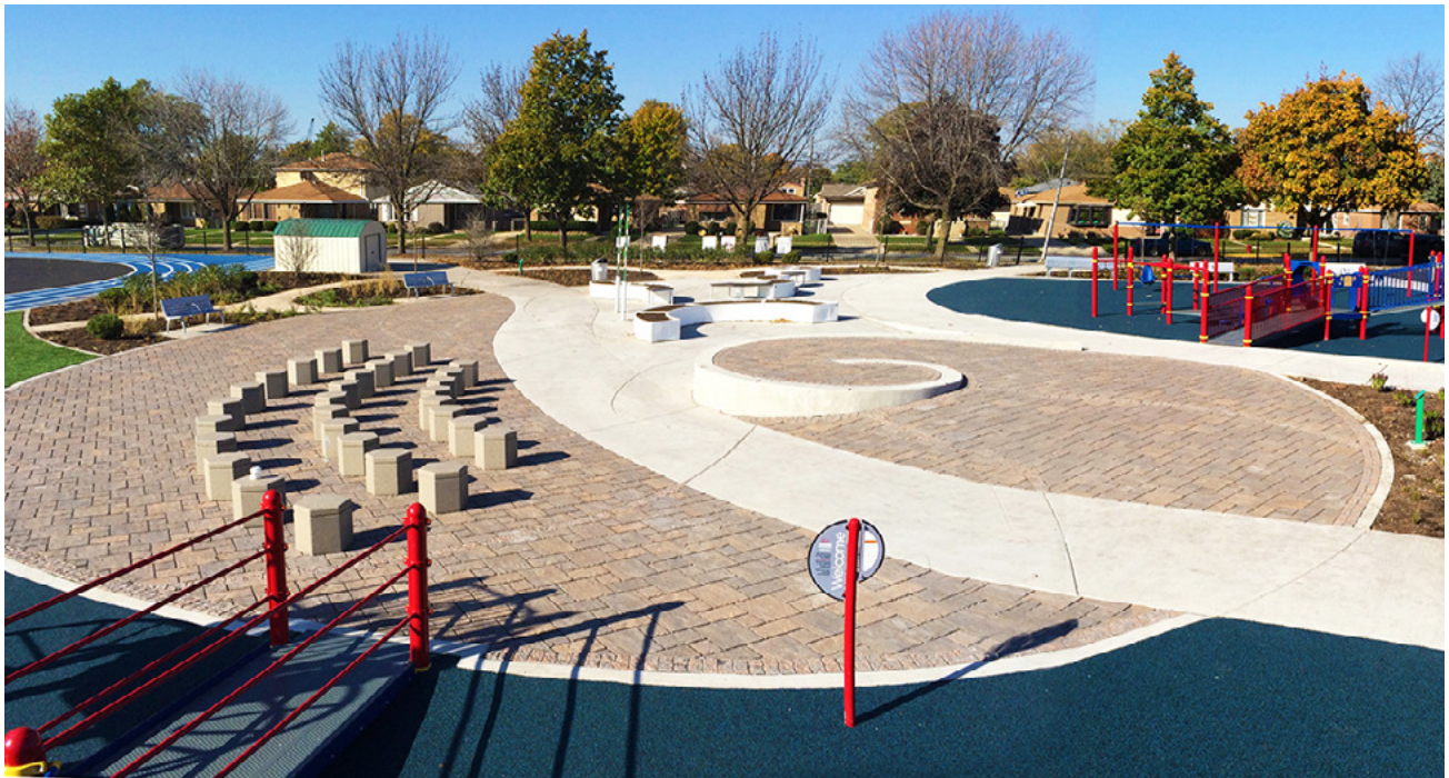
The outdoor classroom is constructed with porous unit paving.
