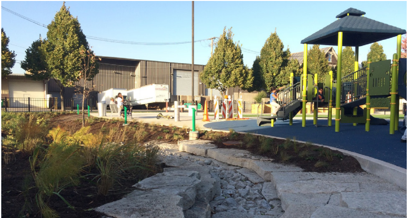
Stepped stone channel directs roof runoff into the bioretention area.
