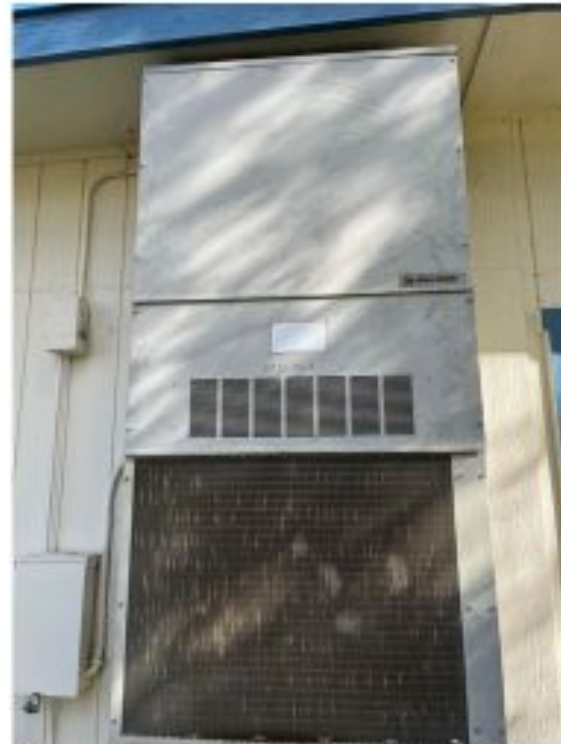
Monta Loma Elementary School, Portables
