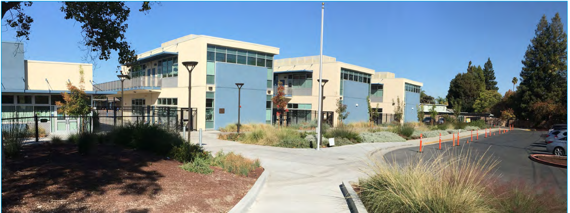
Mariano Castro Elementary School Frontage at Toft Street
