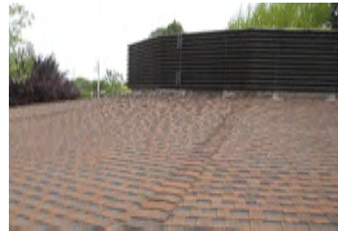
Roof Overview - Building 6
