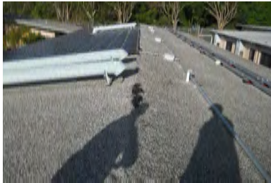
Roof Overview - Building 2
