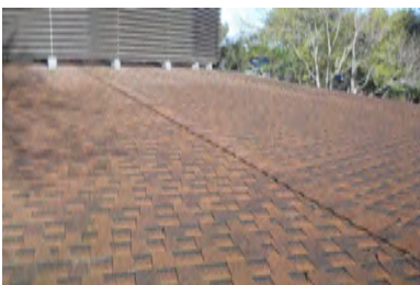
Roof Overview - Building 2
