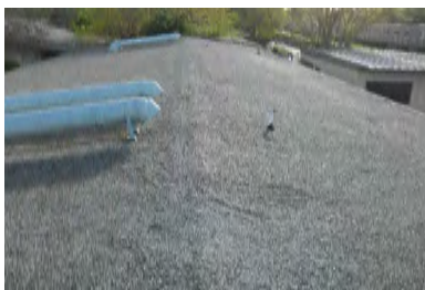
Roof Overview - Building 7
