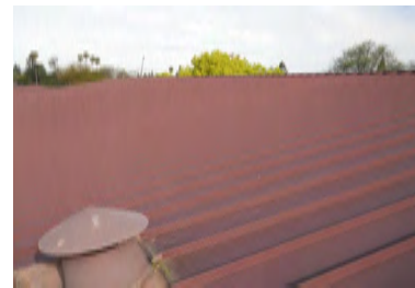
Roof Overview - Building B
