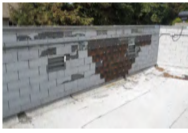
Typical Deficiency - Asphalt shingles are damaged and missing. Recommend replacing.
