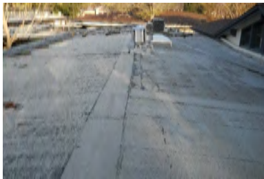
Roof Overview - Building 1
