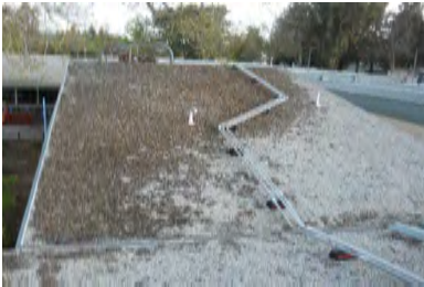
Roof Overview - Building Admin. Office
