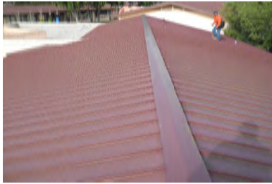
Roof Overview - Building A
