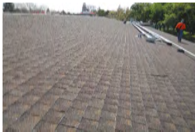
Roof Overview - Building L
