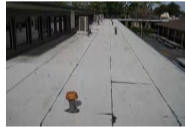
Roof Overview - Building J
