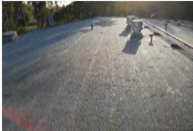
Roof Overview - Building 7
