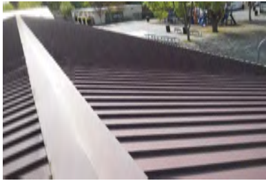
Roof Overview - Building G
