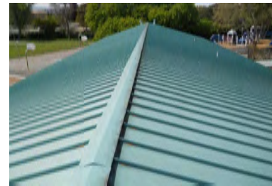
Roof Overview - Building N
