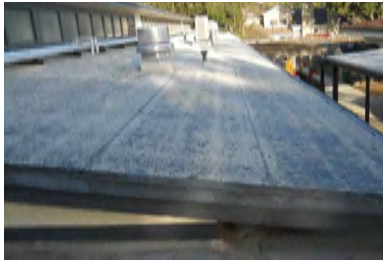
Roof Overview - Building 3 and 4 Similar
