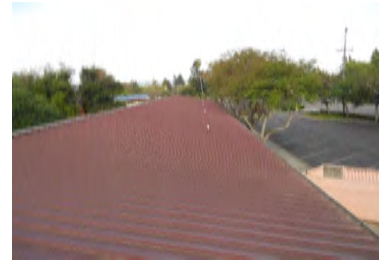
Roof Overview - Building C
