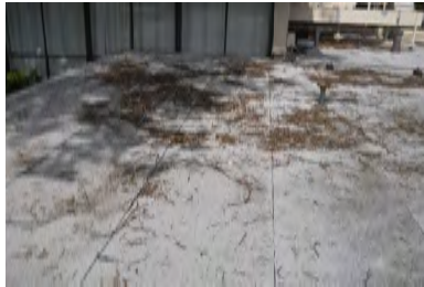
Typical Deficiency - Observed debris at field of roofing. Recommend clearing debris from all gutters, drains, waterways, and field of roof to promote positive drainage.
