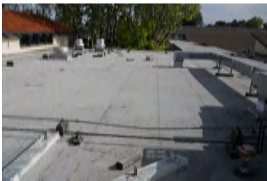
Roof Overview - Building N
