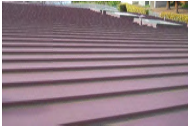
Roof Overview - Building D
