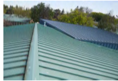
Roof Overview - Building M
