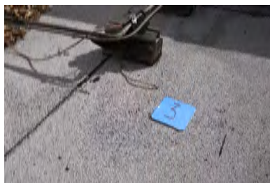
Typical Deficiency - Mineral surfaced cap sheet has blistered. Recommend relief cutting blister, imbed in layer of modified mastic, and apply target sheet of mineral surfaced cap sheet in cold applied adhesive.
