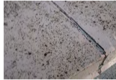
Typical Deficiency - Sealant at coping seams has begun to fail. Recommend removal and replacement of sealant as needed.
