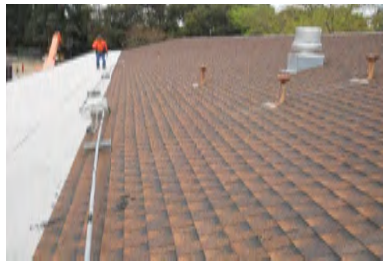
Roof Overview - Building 5
