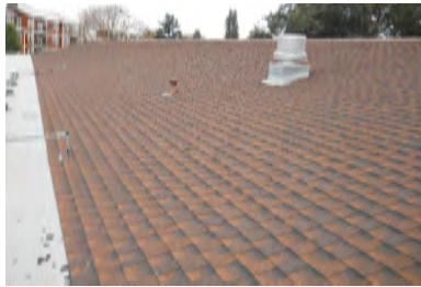
Roof Overview - Building 3
