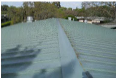
Roof Overview - Building 9
