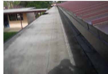
Roof Overview - Building C
