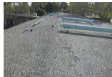
Roof Overview - Building 8
