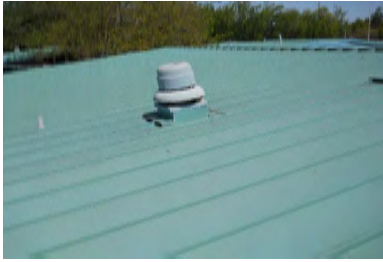
Roof Overview - Building H
