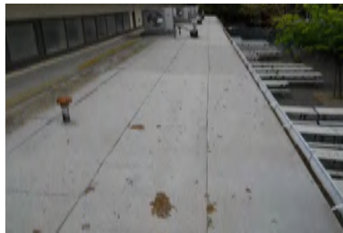
Roof Overview - Building 5
