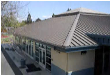
Roof Overview - Building 17
