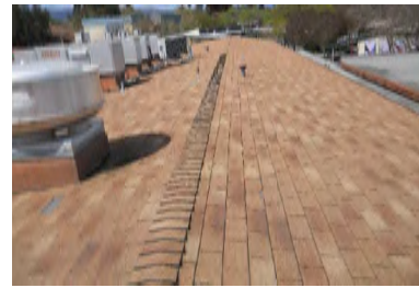
Roof Overview - Building 12
