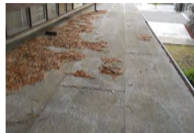
Roof Overview - Building 700
