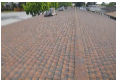
Roof Overview - Building 11
