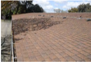
Roof Overview - Building 3 (Building 4&5 Similar)
