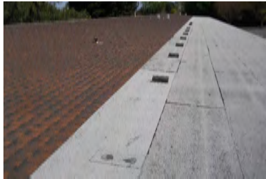
Roof Overview - Building 1
