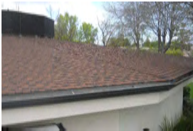
Roof Overview - Building 6
