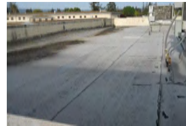
Roof Overview - Building 100
