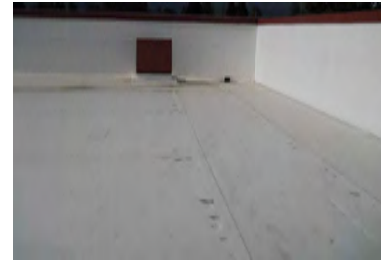
Roof Overview - Building 7B
