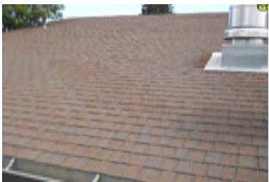
Roof Overview - Building 2
