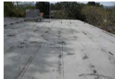
Roof Overview - Building M
