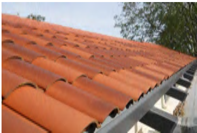
Roof Overview - Building N
