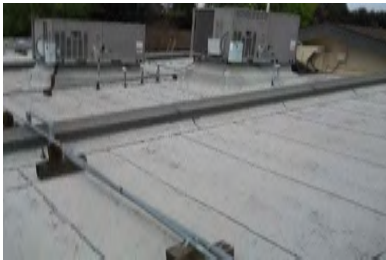
Roof Overview - Building 2 (Building 1, 3, 4, 5, 6 Similar)
