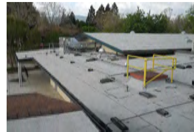
Roof Overview - Building 9
