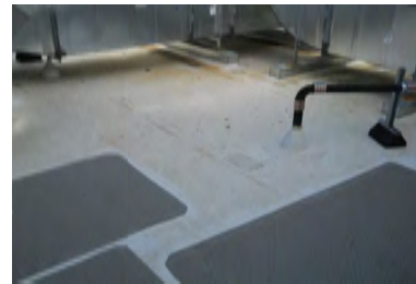
Roof Overview - Building 600
