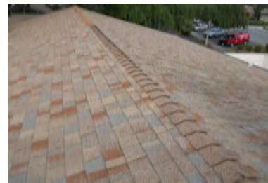
Roof Overview - Building 700
