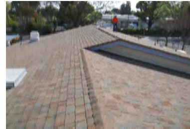
Roof Overview - Building 1000
