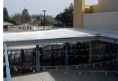
Roof Overview - Building 600
