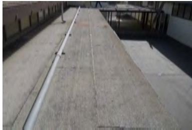
Roof Overview - Building 900
