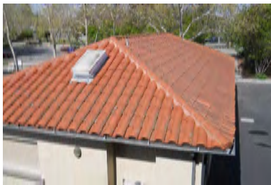
Roof Overview - Building 10
