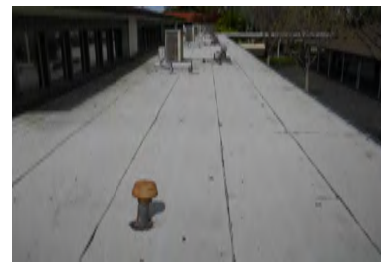
Roof Overview - Building K
