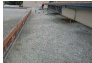
Roof Overview - Building 12
