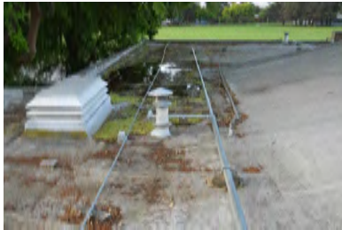
Roof Overview - Building 1
