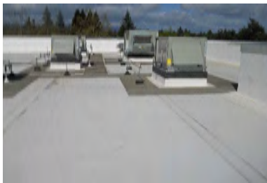
Roof Overview - Building 14
