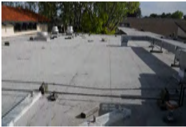
Roof Overview - Building N
