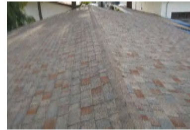
Roof Overview - Building 100
