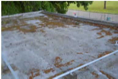
Roof Overview - Building 1
