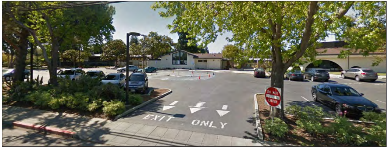
Slater (Google) School Frontage at Gladys Avenue
