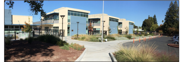
Castro Elementary School
