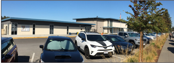
Stevenson Elementary School
