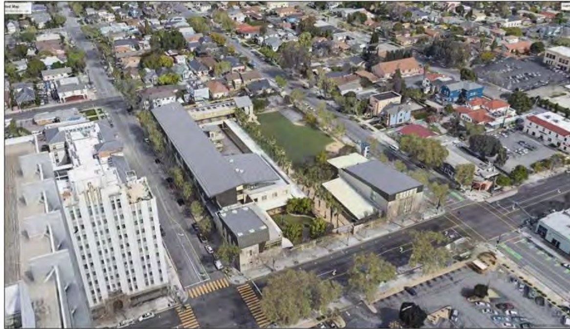
Aerial View over North 6th Street/East Santa Clara Street
