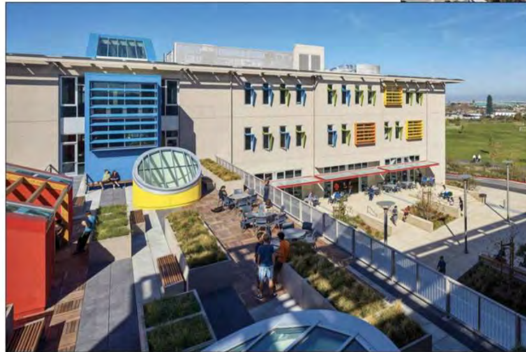
Rooftop Landscaped Terrace on Level 2
