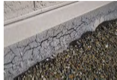
Typical Deficiency - Base flashings show signs of deterioration and cracking. Recommend application of silicone or acrylic coating to maximize usable life of existing built-up roof system.
