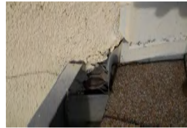
Typical Deficiency - Observed exposed lath and underlayment at roof to wall transition. Recommend stucco patch and as needed sealing to protect underlayment and minimize water intrusion behind stucco.
