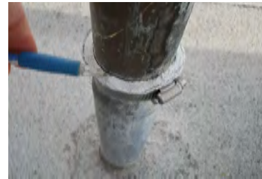
Typical Deficiency - Sealant at lead pipe jacks has begun to pull away from through roof penetration. Recommend replacing sealant as needed, installing stainless steel band clamps, and storm collar.
