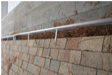
Typical Deficiency - Gutter brackets have been face fastened through asphalt shingle. Recommend removal and repositioning bracket. Repair asphalt shingles as needed. Typical Deficiency - Gutters are full of debris. Recommend clearing debris from all gutters, drains, waterways, and field of roof to promote positive drainage.
