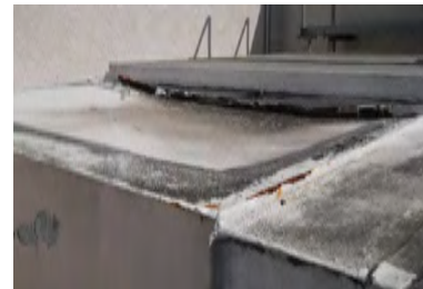
Typical Deficiency - Mechanical duct work damaged and deteriorated. Recommend replacement of damaged duct by licensed mechanical contractor and coating with acceptable silicone or acrylic coating.
