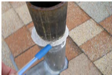
Typical Deficiency - Pipe jack sealant has begun to pull away from through roof pipe penetration. Recommend application of flexible flashing self-adhered tape and or sealant, and install storm collar.
