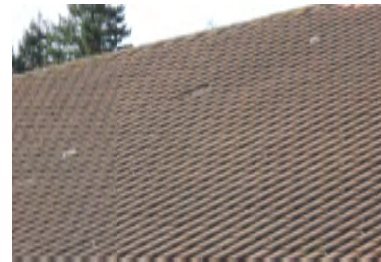
Typical Deficiency - Missing concrete S tile. Recommend replacement of all missing and or damaged tiles.
