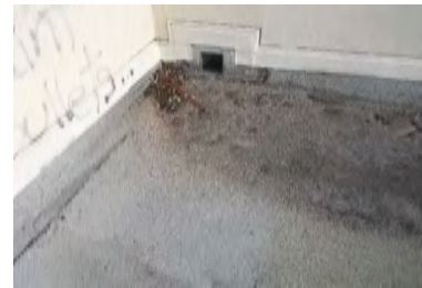
Typical Deficiency - Through wall scuppers should have debris screens. Recommend installation of gutter screens to promote positive drainage.
