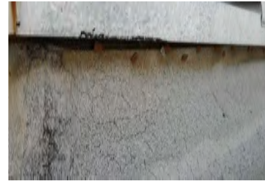
Typical Deficiency - Base flashing at mechanical curb has not been properly skirt flashed. Recommend installation of GSM skirt flashing.
