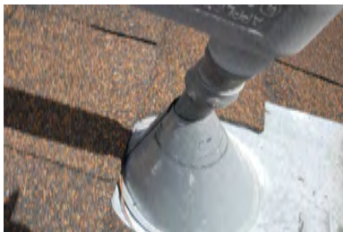
Typical Deficiency - Pipe jacks are missing sealant and or flexible self- adhered flashing tape. Recommend sealing, and install storm collar.
