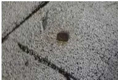
Typical Deficiency - Observed fastener penetrating through finished built-up roofing. Recommend removal and patch.
