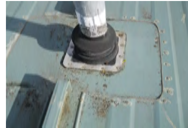
Typical Deficiency - Detailing at through roof penetrations show signs of cracking and delamination. Recommend touch up of sealants..
