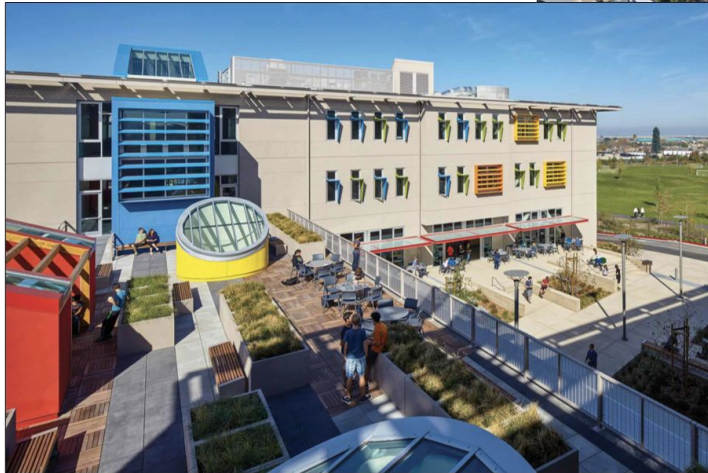
Rooftop Landscaped Terrace on Level 2
