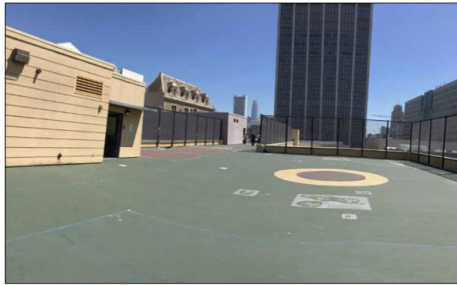
Rooftop Play Area at Level 4 with Storage and Stairs
