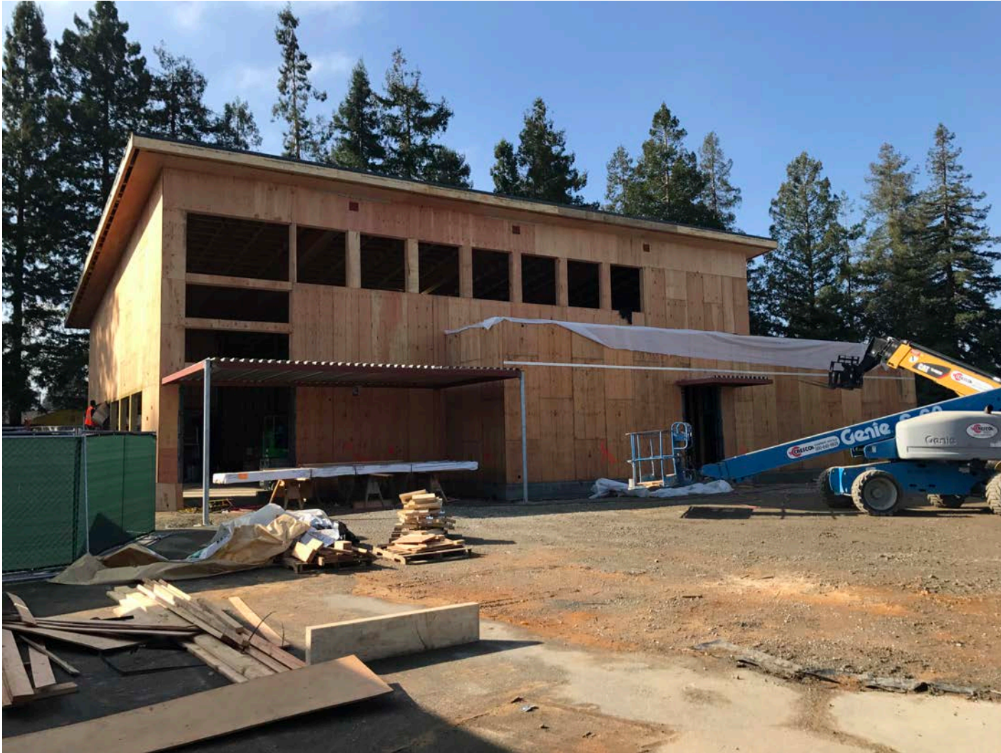
Landels Elementary School – New MUR
