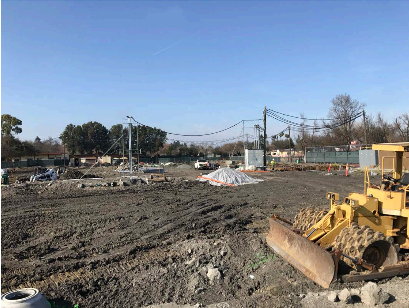
Stevenson Elementary School – Building Pad
