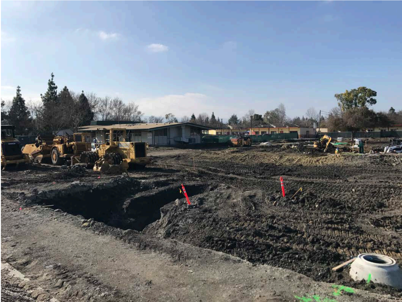
Stevenson Elementary School – Foundation pad
