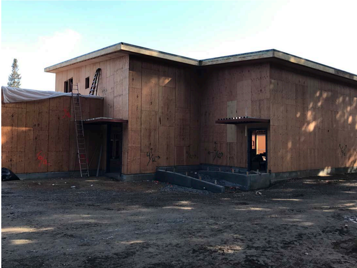
Huff Elementary School – MUR Stage Door
